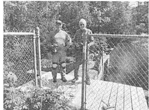
Dam Committee Members Complete Decking
